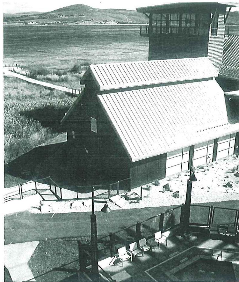
Above: The Swaner EcoCenter's Education Center sits adjacent to Newpark Hotel's swim-out pool and paved trail and expects to achieve LEED Platinum certification.
